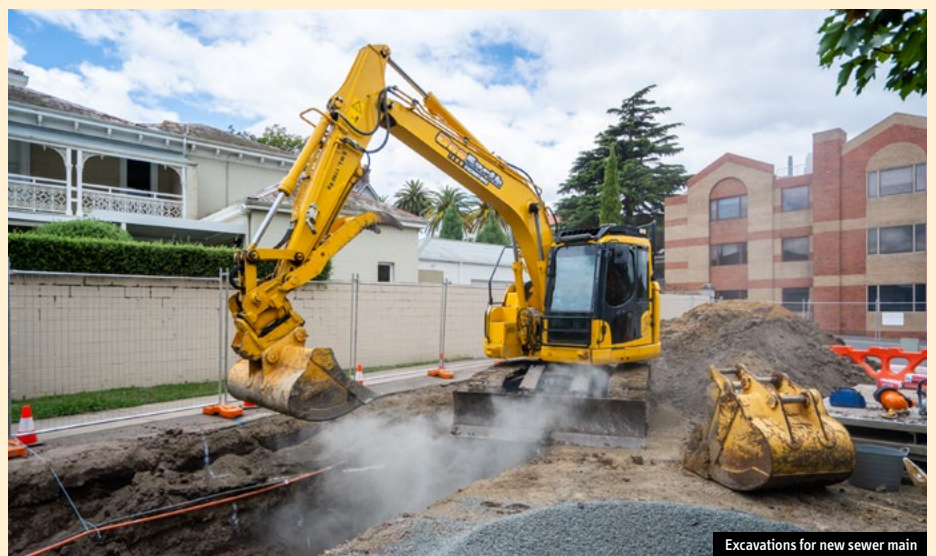
Excavations for new sewer main
