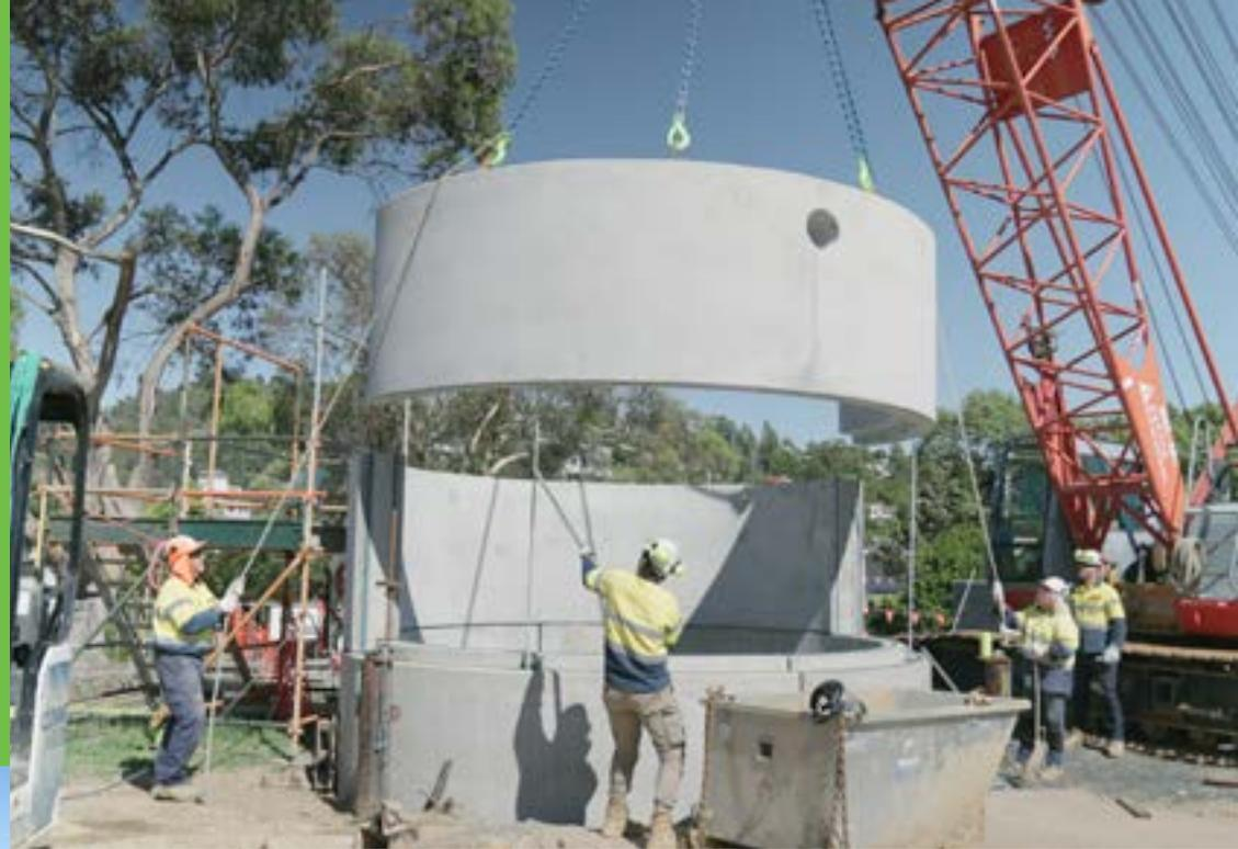
Precast concrete segment lifted into place for the new under-ground diversion chamber at our Margaret Street Pump Station.
